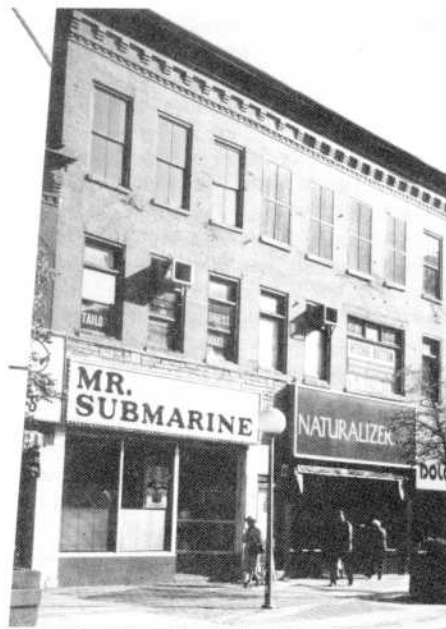
The "Canadian Block" in 1986, located on the northwest corner of King & Ontario streets in Kitchener.
